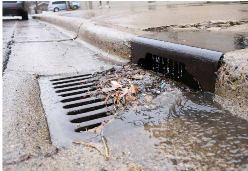
Stormwater runoff flowing into a storm drain.
