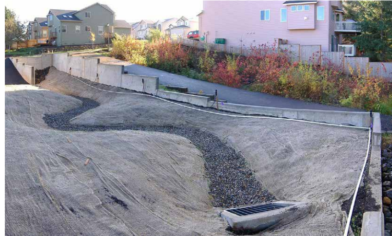
A bioswale under construction.
