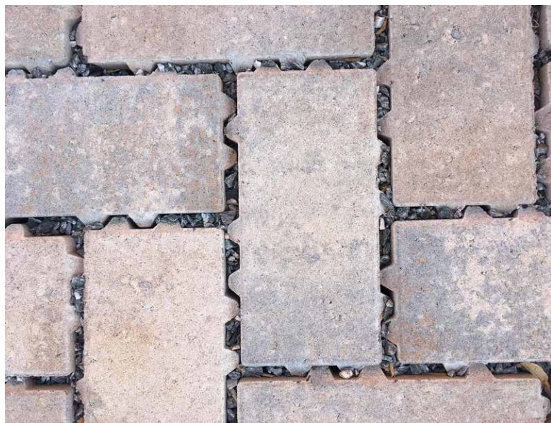
Permeable pavers allow water to soak into the ground, reducing runoff.
